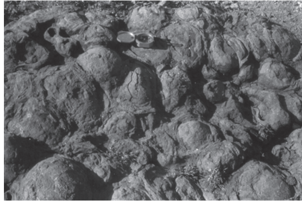
Fig.6.4 : Exfoliation (Flaking) and granular disintegration
