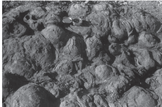
Fig.6.4 : Exfoliation (Flaking) and granular disintegration
