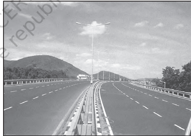
Fig. 8.3 : Dharmavaram Tuni National Highway, India
