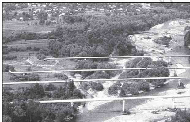
Fig. 8.17: Pipelines transporting natural gas in Ukraine
