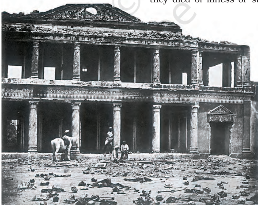
Fig. 10.9 Secundrah Bagh, Lucknow, photograph by Felice Beato, 1858
