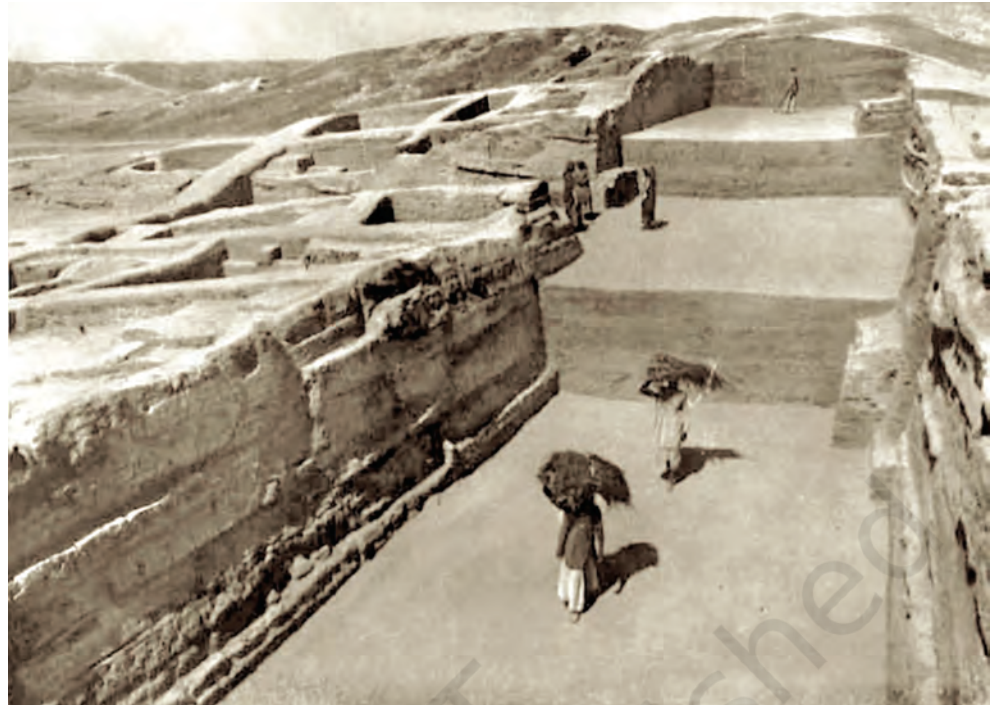
(Top) Fig. 6.4. A wide street at Kalibangan (Rajasthan), in the lower town area.
