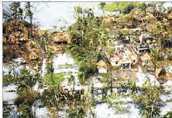
Destruction caused by a cyclone
