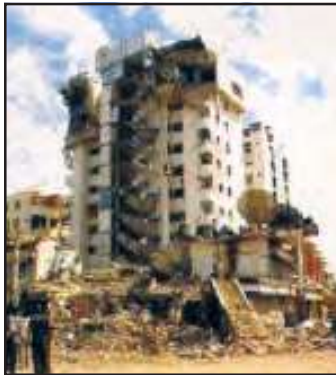
Fig. 3.3a: Destruction caused by an Earthquake in Gujarat
