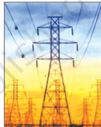
Fig. 3.7: National Power Grid to supply Electricity
