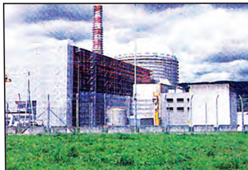
Fig. 3.16 : Nuclear power station, Kalpakkam
